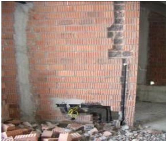
Services Chasing / Repair
